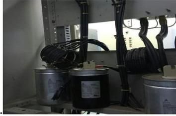
Gambar. 5. Kapasitor Bank SIEMENS di Intake Karang Anyar
