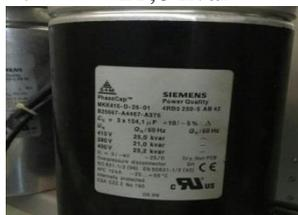
Gambar. 4. Nameplate Kapasitor Bank di Intake Karang Anyar
