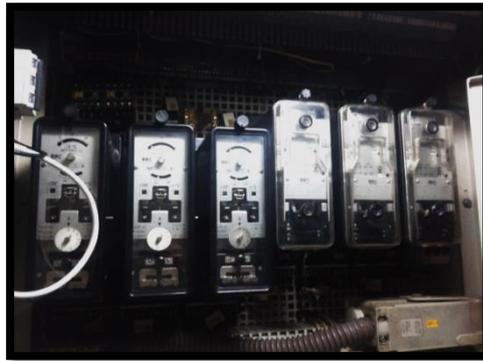
Gambar 1. Relay Tipe STKK dan ISM di Panel 20 kV MSS <sup>[1,2]</sup>
